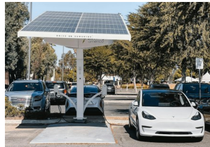
RES for EV charging
